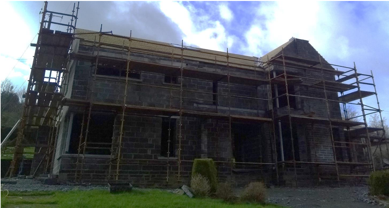
Roof Before Slate Finishes
