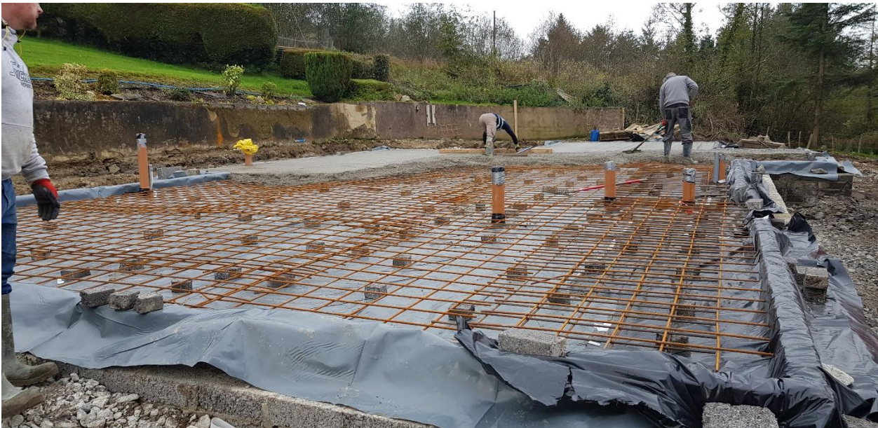
Steel Reinforcement and Shuttering to Wet-Cast Concrete Slab
